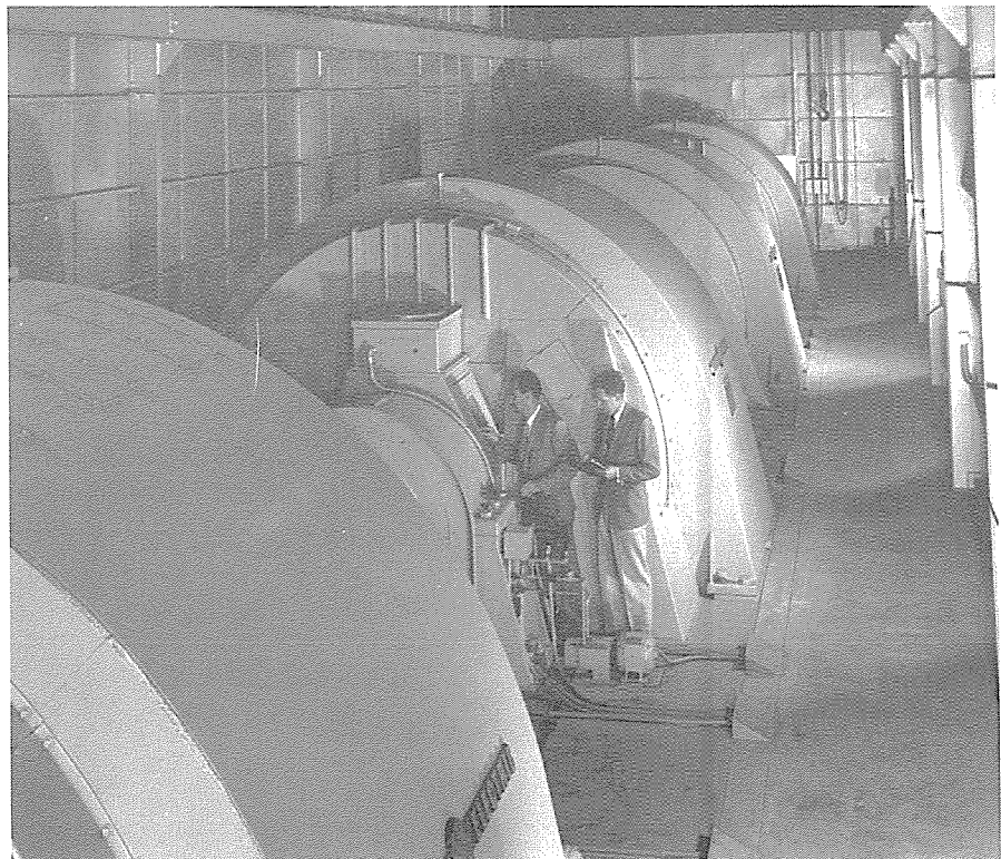
45,000 horsepower main drive motors for the Unitary Plan Wind Tunnel.
