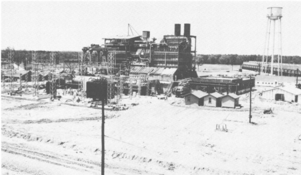
General view of Greens Bayou No. 1 (right) & No. 2, with the 66 KV switchyard in the foreground and cooling towers in the background.
