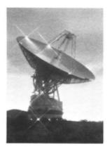
ABOVE: THIS DEEP SPACE NETWORK ANTENNAIN CALIFORNIA'S MOJAVE DESERT, SHOWN IN ITS 64-METER-DIAMETER CONFIGURATION, WAS EN-LARGED TO 70 METERS TO SUPPORT THE VOYAGER NEPTUNE ENCOUNTER.
