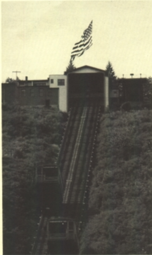
An Uphill view of the Incline.
