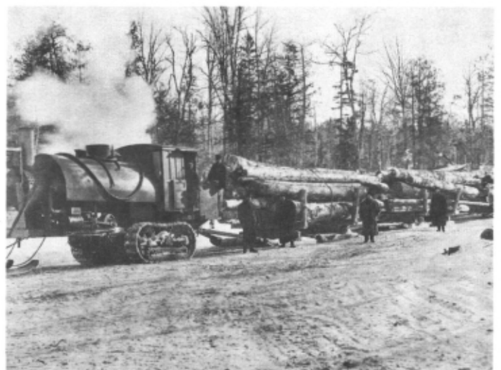
There were no brakes on a log hauler or on its train of sleds...nearly every road had its downgrade that made steerers pray that should they live this once more then they would find some other way to make a living."—Yankee Magazine, March 1965.
