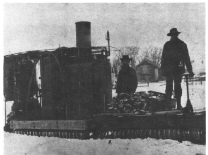
A Peavey Log Hauler, Traction was obtained by revolving screws.
