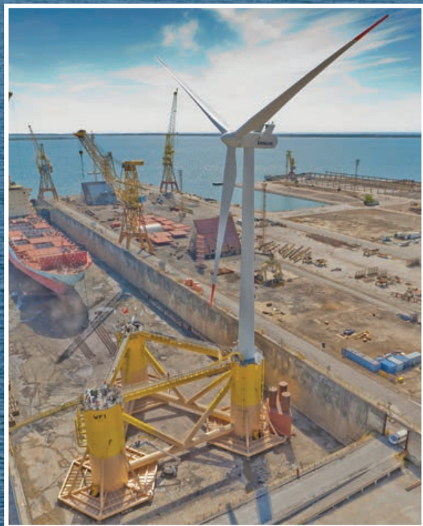
A prototype of a WindFloat platform tested offshore was built in drydock at the Lisnave facility (inset) near Setubal, Portugal.
